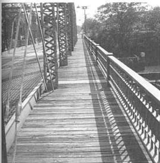
The Bridge Monument Showing Wooden Sidewalks. (Photo: Robert Smithson.)
